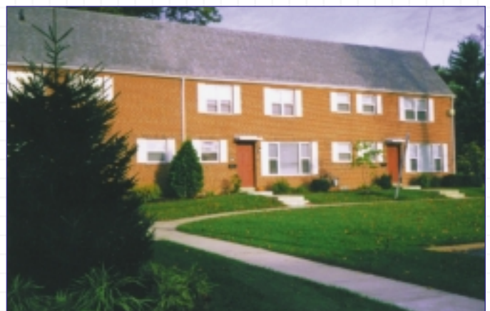
A close-up of one of the 56 buildings located on the property.
